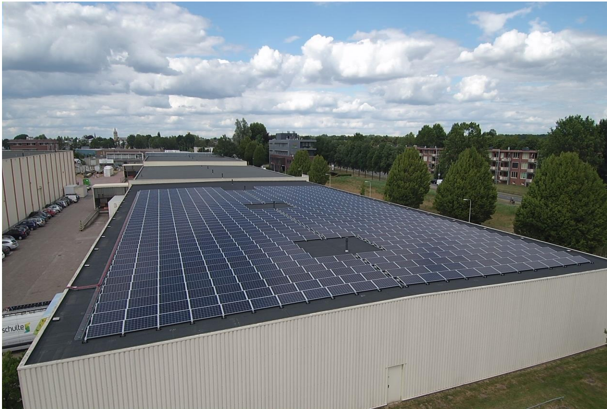
Project Shelter Storage
